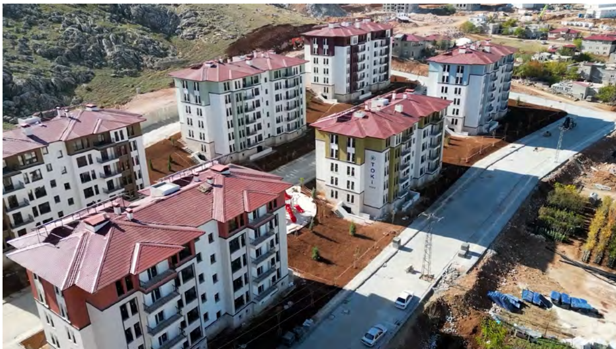
Minister Özhasseki shared photos of disaster residences under construction. Mehmet Özhasseki, Minister of Environment, Urbanisation, and Climate Change, shared photographs showing the final state of the houses under construction by the Mass Housing Administration (TOKİ) in Kahramanmaraş after the earthquakes that occurred on February 6.) (ÇŞİDB - Anadolu Agency)
