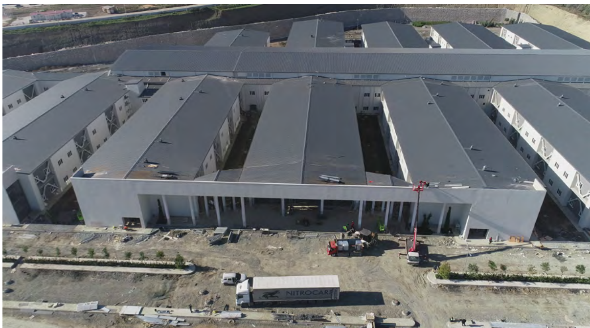
The construction of the 400-bed Antakya Training and Research Hospital, which commenced on March 24 in Hatay, centered in Kahramanmaraş and affected by the earthquakes of February 6, has reached the completion stage. The construction work of the hospital, established on an area of 122 thousand square meters, 57 thousand square meters of which is closed, in the Gülderen District of the Central Antakya district, continues without slowing down. (Ozkan Bilgin - Anadolu Agency)
