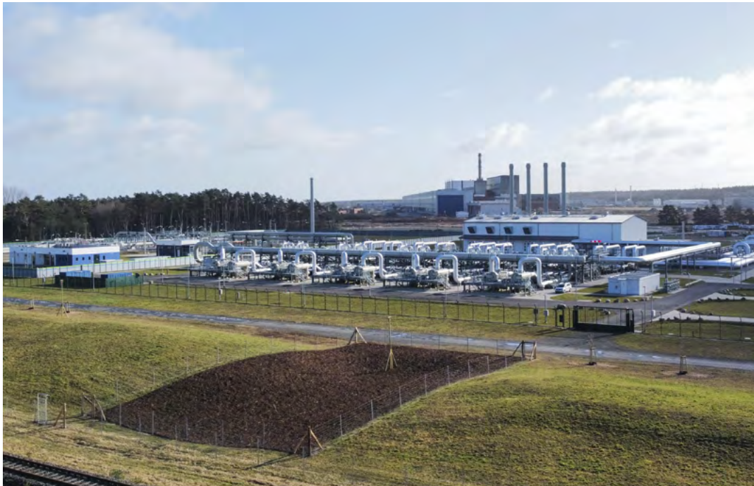
A view of Nord Stream 2 gas receiving station on Germany's Baltic coast in Lubmin on February 23, 2022. Germany halted the Nord Stream 2 pipeline project after Russia's War on Ukraine. (Abdulhamid Hoşbaş - Anadolu Agency)
