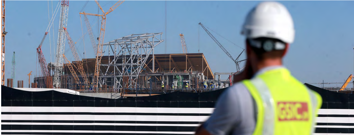
Construction workers are seen outside the construction site of the Al Bayt Stadium in Al Khor, Qatar on June 20, 2017. The stadium will be a venue for the FIFA World Cup 2022. (Mohamed Farag - Anadolu Agency)
