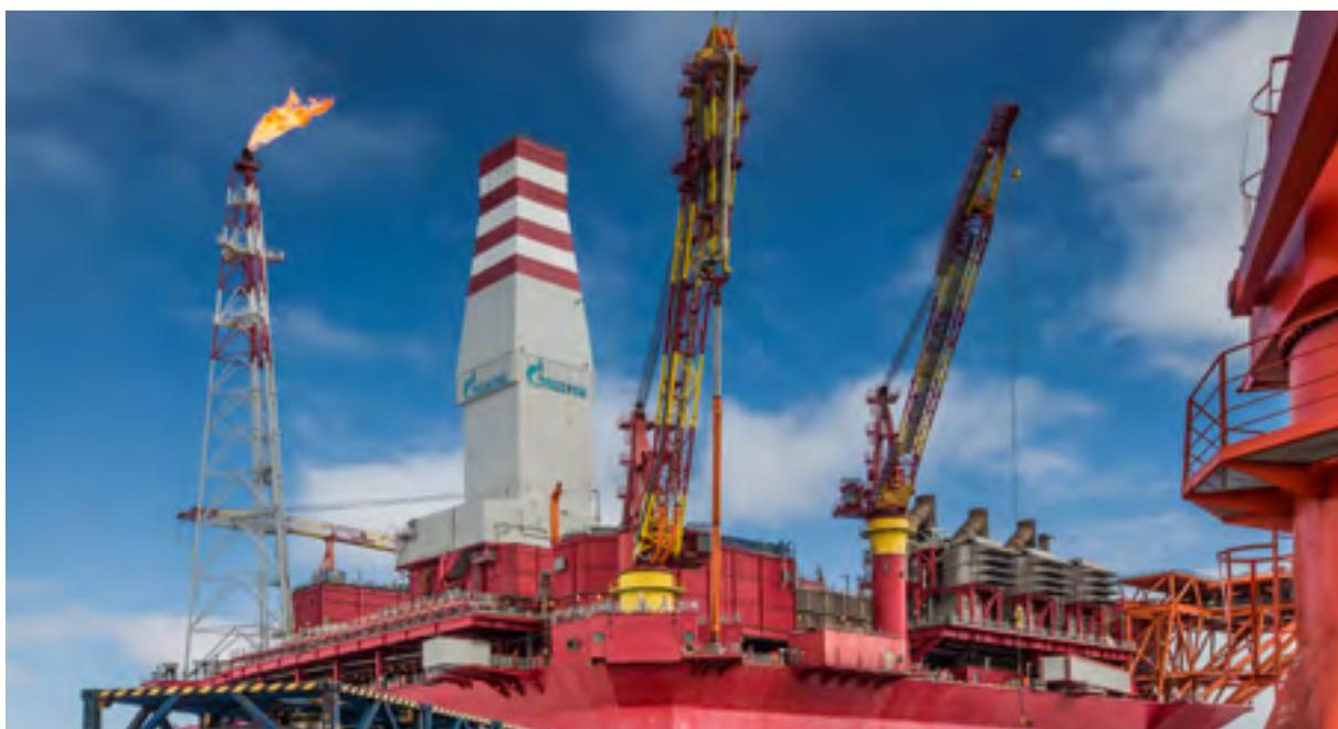
*The Prirazlomnaya offshore ice-resistant oil-producing platform is seen in the Pechora Sea, Russia on May 8, 2016. Prirazlomnaya is the world's first operational Arctic rig that can process oil drilling, production and storage, as well as end product processing and loading.*
