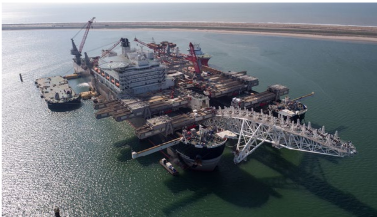
Pioneering Spirit is seen at the construction site of TurkStream and Russian company Gazprom gas pipeline's offshore of Anapa city in the Black Sea on June 23, 2017. Construction is run with the world's largest construction vessel Pioneering Spirit with the length of 382 meters and width of 124 meters. Pioneering Spirit departed from Port of Rotterdam. TurkStream will directly connect the large gas reserves in Russia to the Turkish gas transportation network, creating a reliable source of energy for Turkey and south-east Europe as construction of the project began today.
